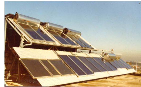
Large outdoor test laboratory for solar thermal energy products
