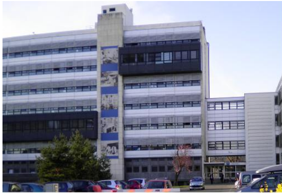
MATEIS building in INSA-Lyon
