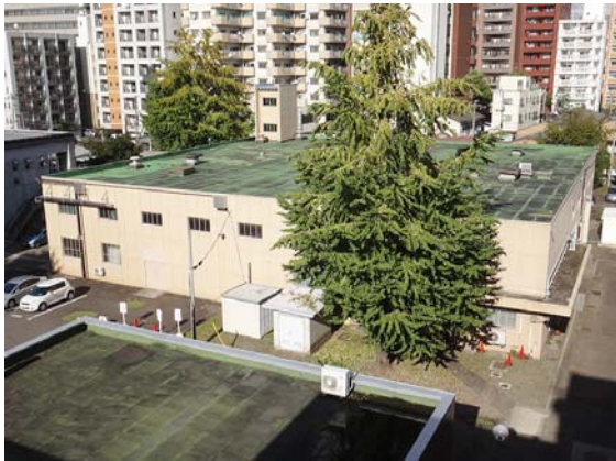
高速流実験棟 High-speed flow experiment building
